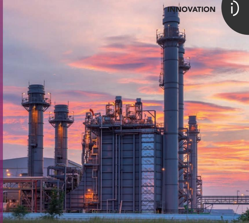
**Advanced Ultra Supercritical (AUSC) materials are subject to severe conditions in terms of service requirements (temperatures around 700 °C, pressures around 36.5 MPa) and environment (high chlorine and sulfur environments during the whole life cycle of the power plant).**
